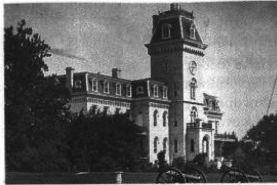
ca. 1872 - In 1868 the building camouflaged its expansion upward with a fashionable Second Empire mansard roof. The tower also grew higher and acquired a water tank.
