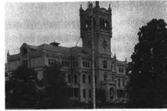
ca. 1910 - In 1884 and 1887 the rear of the building was expanded in a Gothic Revival style, and in 1890 the front of the building caught up, growing still higher in the process. The building has housed veterans from every American war since the War of 1812.
